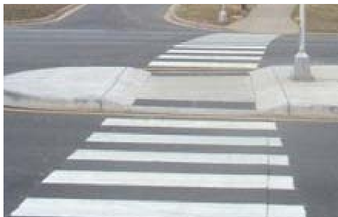
Example of improved pedestrian crossing visibility
